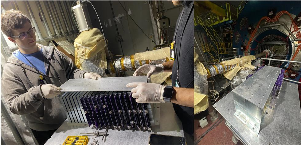
FIG. 6. The generation 2 CALI prototype being installed in the East platform of STAR (left), facing the IP with minimal material obstructing it (right).
